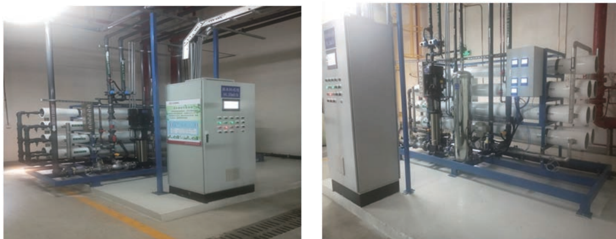
Concentrated water recycling system of the semi-conductor business division
