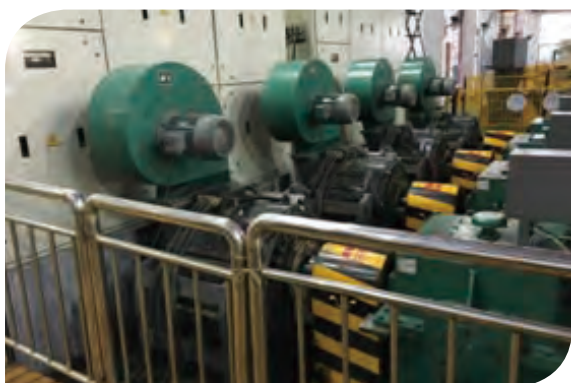
Before Alternation: 4,000 rpm with an average noise of 93dB.
