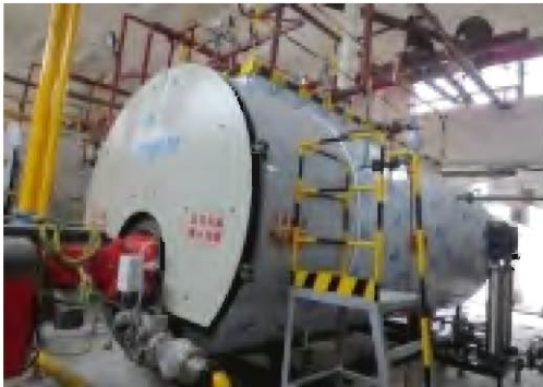
The newly built gas-fired boiler
