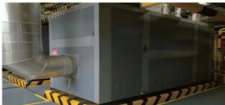
Upgrade of boilers and air-conditioning systems
